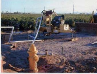
Direct connection from hydrant to pump.
