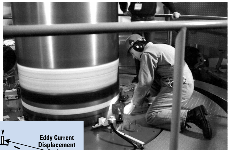
Figure 5 Installing the Probes A B.C. Hydro employee installs the displacement probes on the turbine guide bearing.
