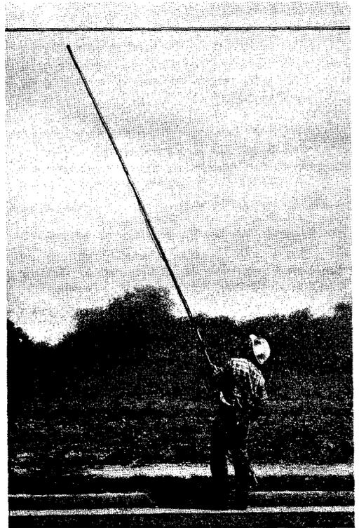
Fig. 19—Locating a Leak Using Wand or Pole Probe Method
