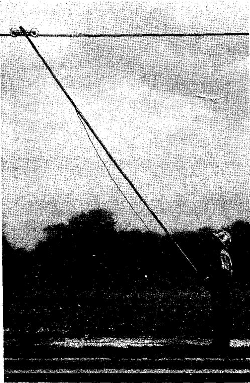
Fig. 18—Locating a Leak Using Trolley Method
