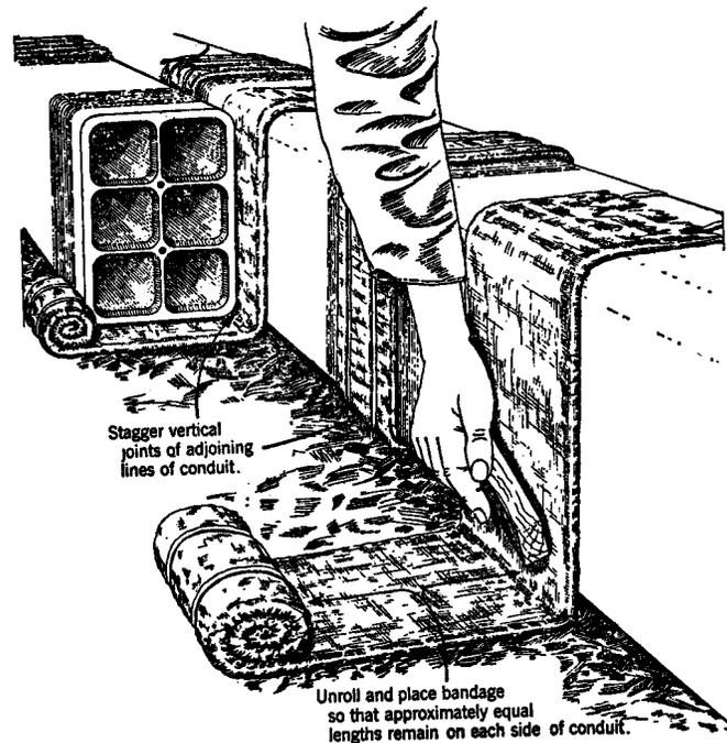
Figure 15-17 - Underground Mortar Bandage
