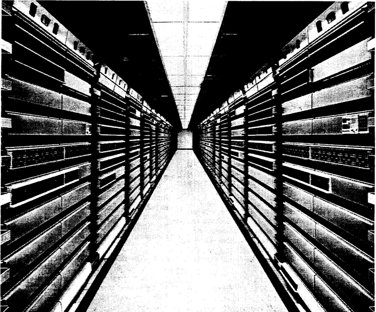
**Figure 3—*COSMIC* Distributing Frame Installation**
