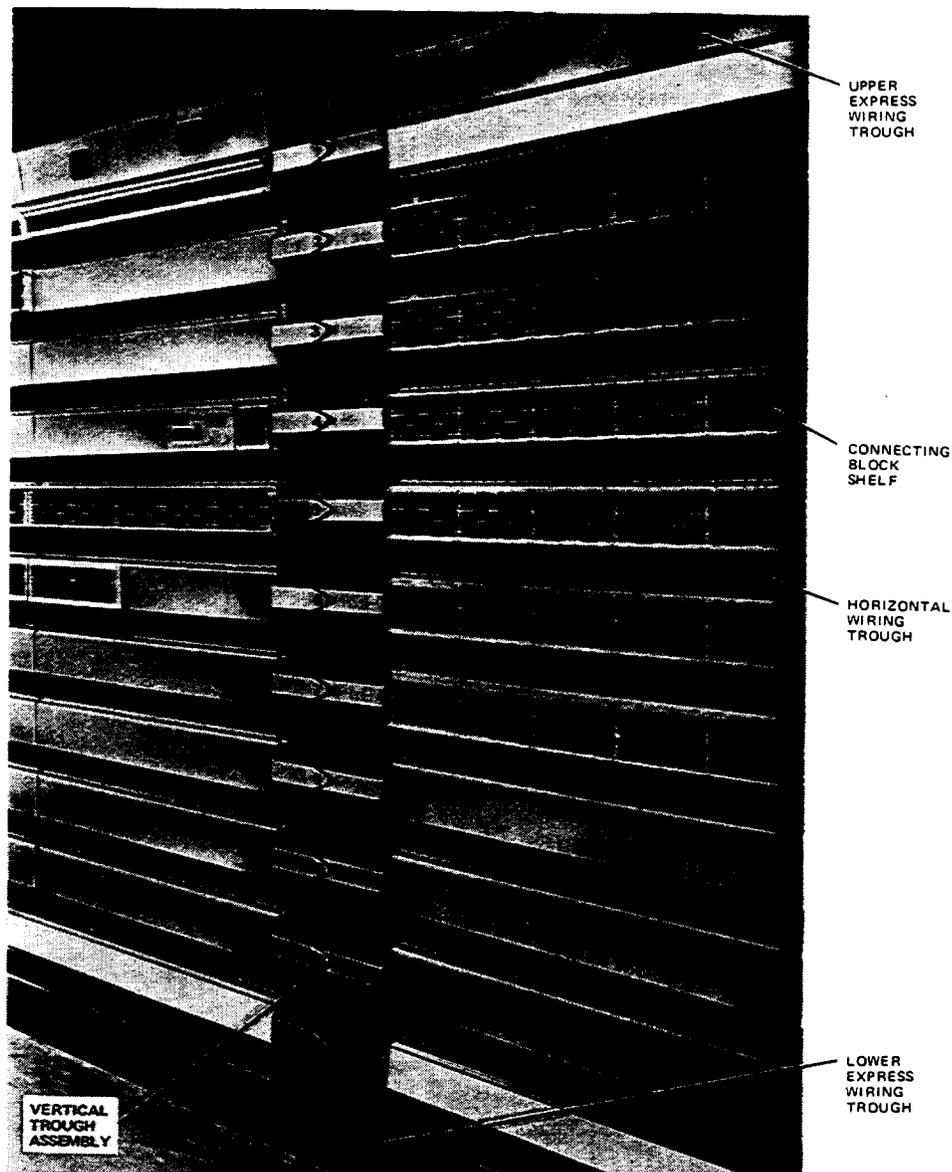
Figure 4—Typical *COSMIC*-Type Distributing Frame (Front View)
