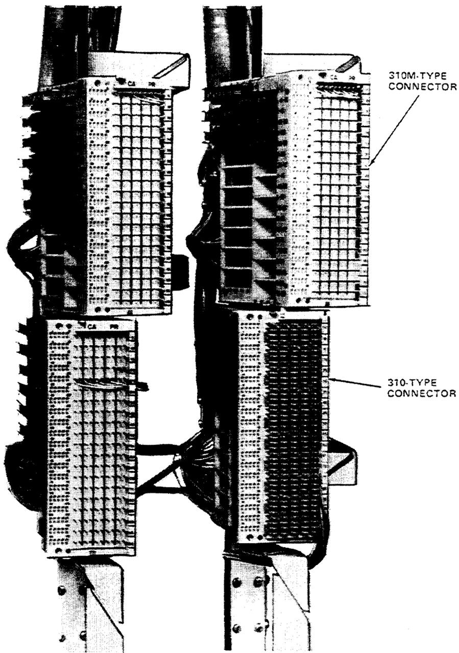
Figure 19—310M Connector (Extends 7 Inches From Face of Vertical Frame Mounting Bar at a 12.5-Degree Angle)
