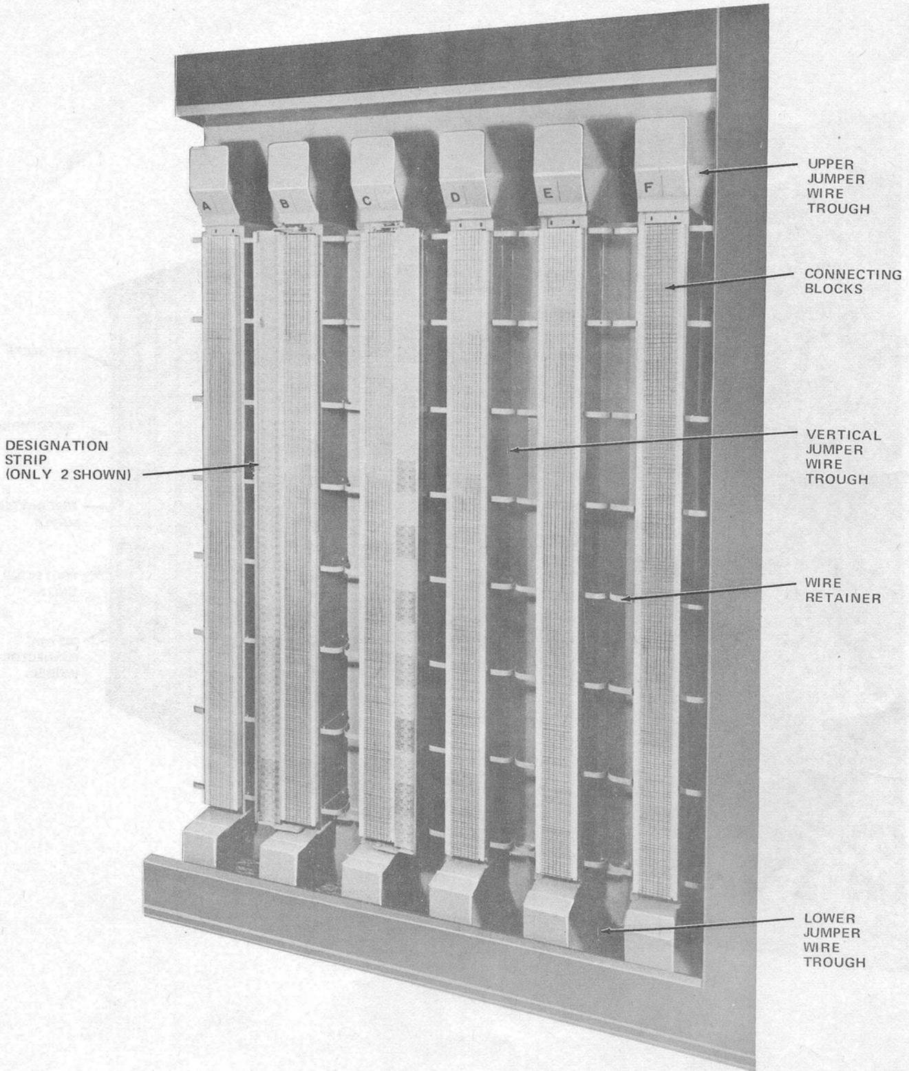
Fig. 3—Trunk Distributing Frame (or Intermediate Distributing Frame)
