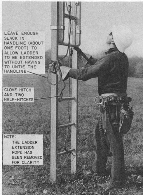
**Fig. 20—Method of Securing Handline**
