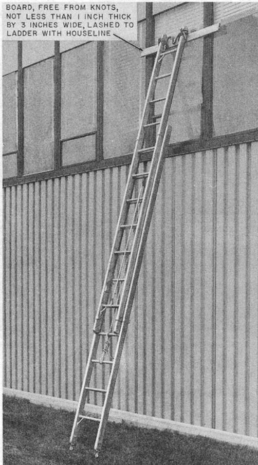
**Fig. 16—Ladder Placed in Front of Window**
