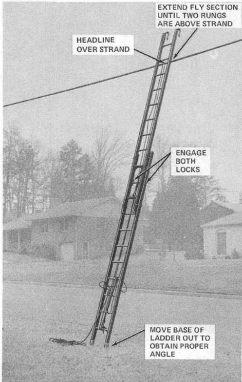
Fig. 21—Ladder in Working Position
