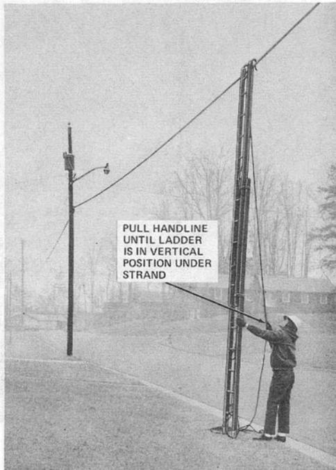
Fig. 19—Ladder in Vertical Position
