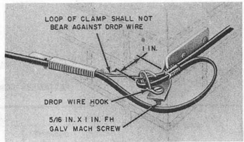
Fig. 7—First Attachment, Corner Bracket
