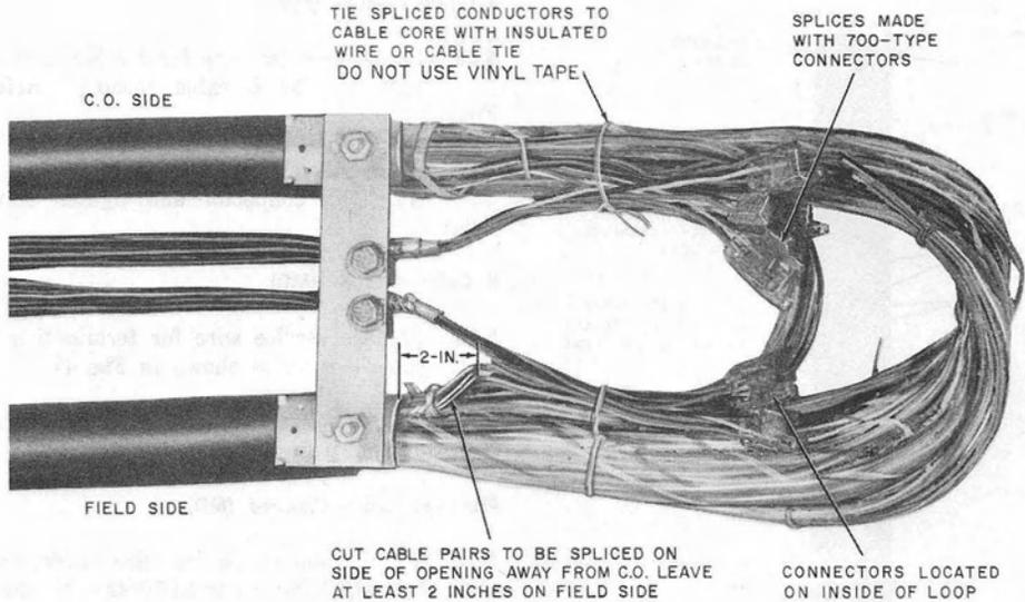
Fig. 6—Wire Work Completed—14-Type Closure
