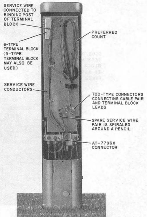
Fig. 11—Service Wires Terminated in PC6/48 Cable Closure—Preferred Count Mode
