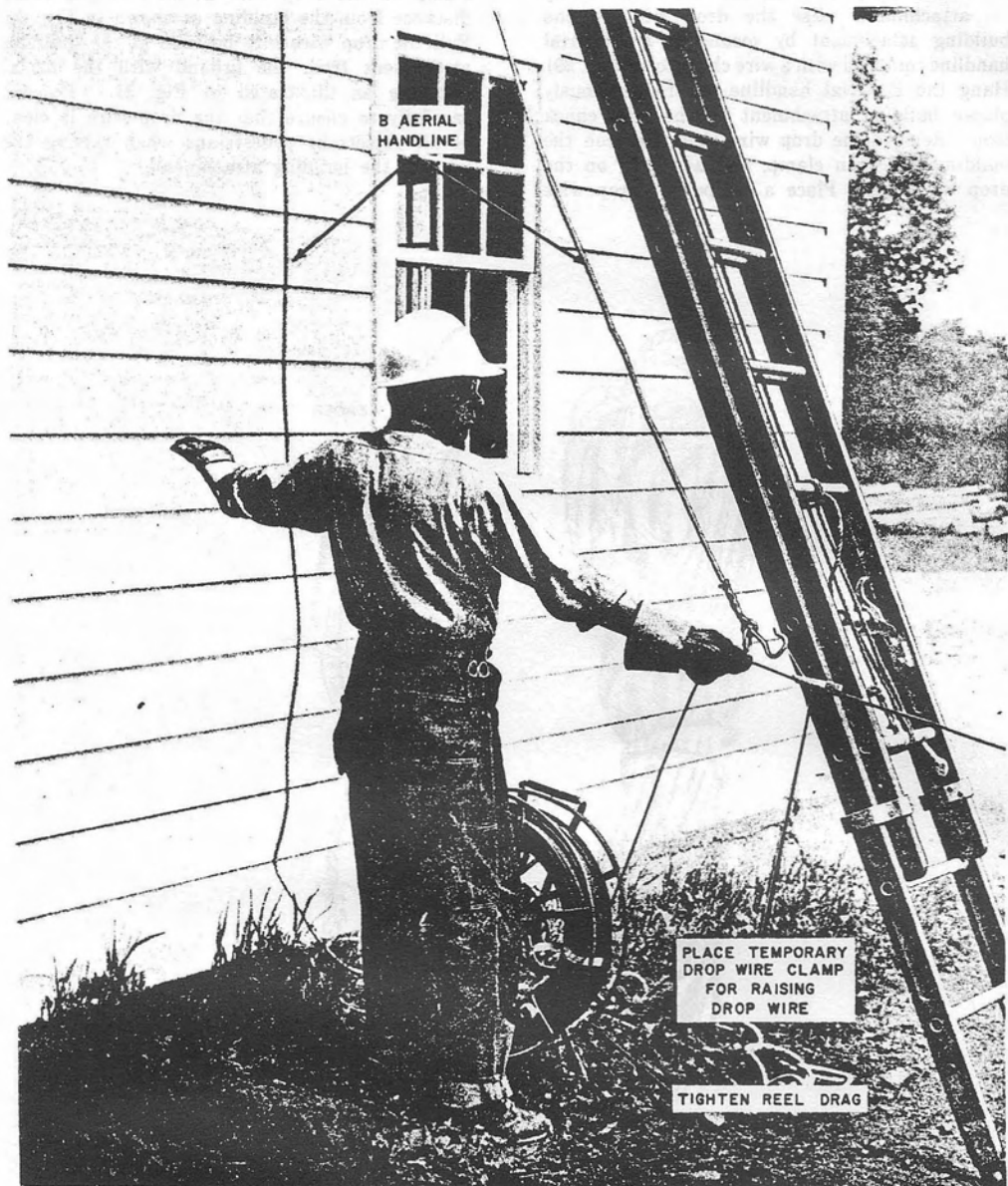
Fig. 30—Locating Temporary Drop Wire Clamp
