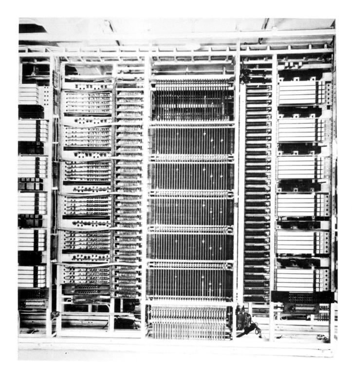
Figure 5-1 Typical Panel Dial Selector Frame
