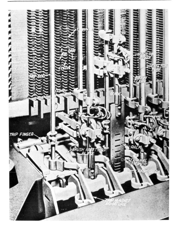
Figure 5-4 Panel Type Selecting Mechanism
