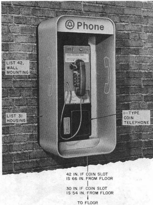
**Fig. 3—List 31 Housing—Wall Mounted (List 4 Arrangement)**
