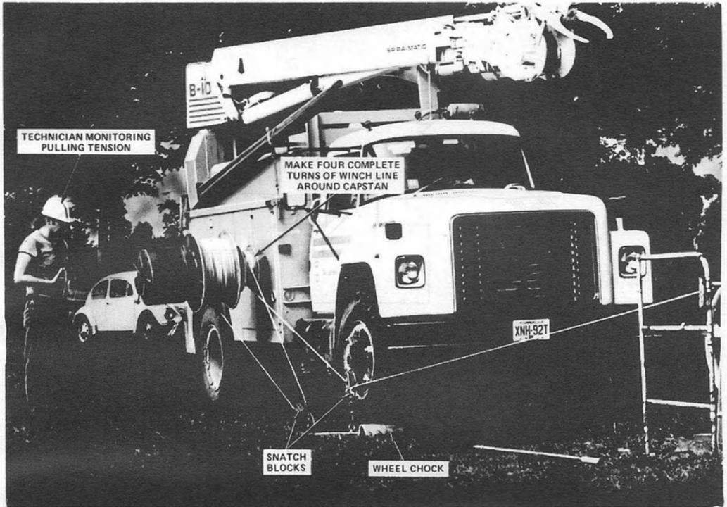
Fig. 8—Pulling Truck Set Up at Manhole
