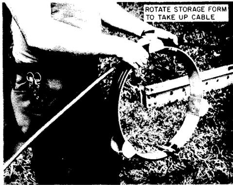
**Fig. 14—Excess Cable Being Coiled on Storage Form**
