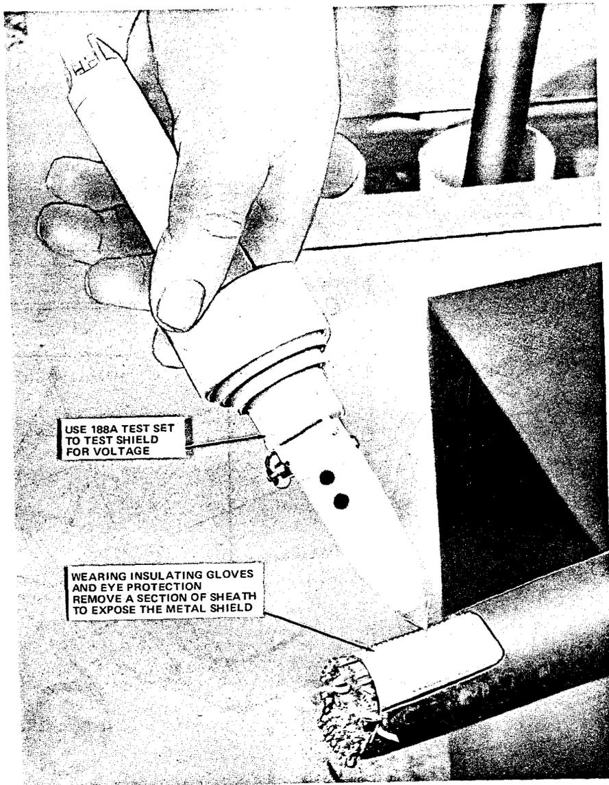
Fig. 1—Testing Cable Sheath for Voltage
