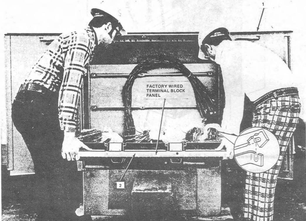
Step 13—Installation of Frame Equipped With Terminal Block
