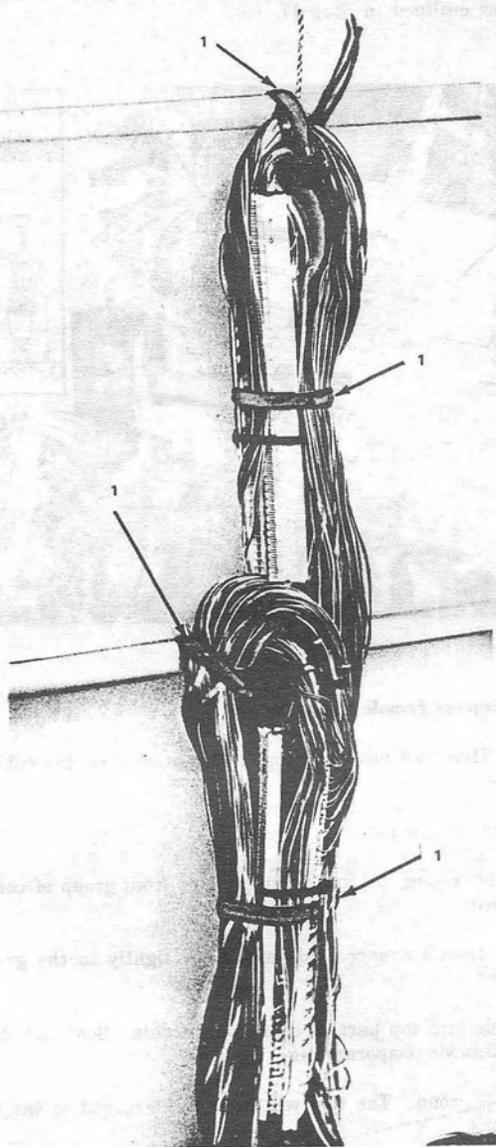
**Step 16—Spliced Groups Secured to Splicing Support**
