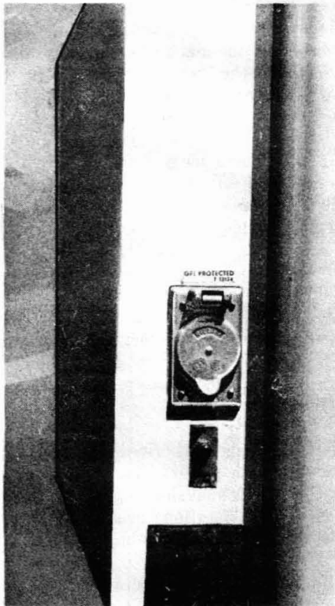
Fig. 8—Electrical Outlet With GFI Protection
