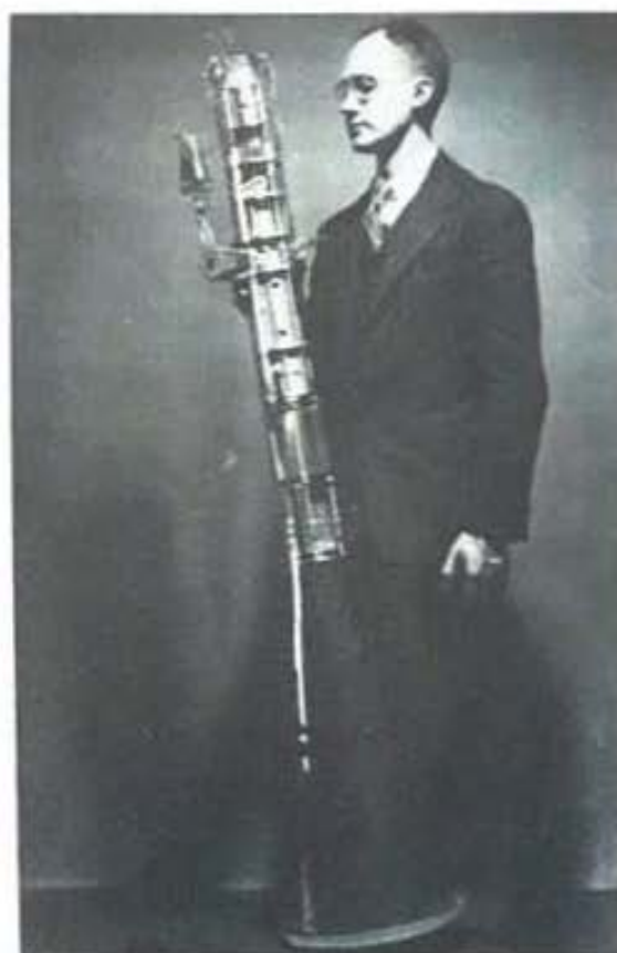
Fig. 3-9. C. J. Calbick with the picture tube designed for television demonstrations by C. J. Davisson. The tube was extremely long to avoid raster distortion.
