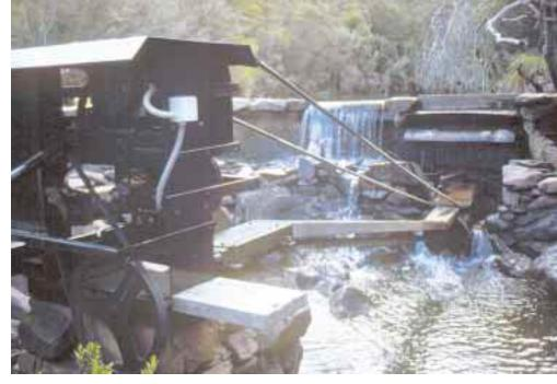
Above: An upstream view of the hydro installation and the 1.2 meter high weir. The "power tower" in the foreground houses the alternator and pump.
