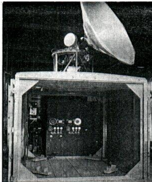
The original model, developed and built in the Radiation Laboratory in 1941 and known as XT-1. This was the first radar capable of following a target automatically without human aid
