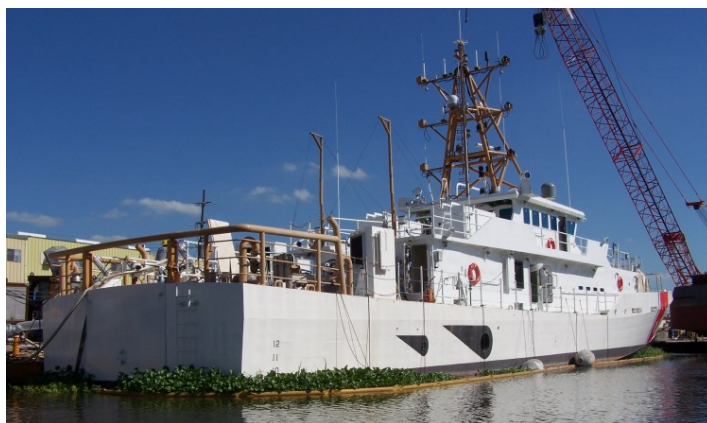
FRC Construction in Lockport, LA
