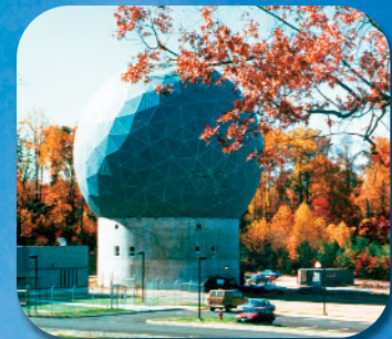
100-ft (30.6m) diameter MSF radome
