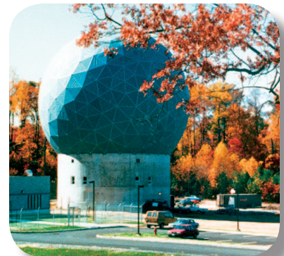
100-ft. (30.6m) diameter MSF radome.
