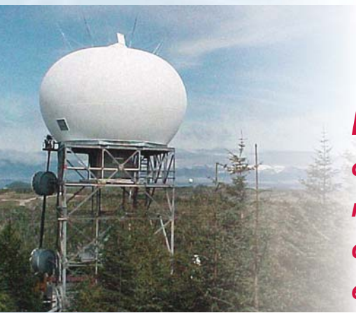
35-ft. (10.7m) diameter oblate radome for digital air surveillance radar application
