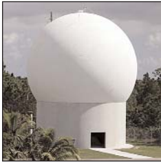
57-ft. (17.4m) sandwich radome – weather
