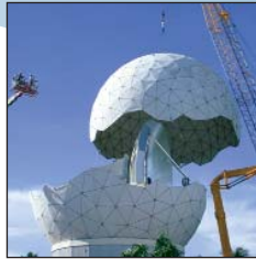
68-ft. (20.8m) metal space frame radome top cap lift
