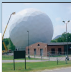
93-ft. (28.3 m) metal space radome undergoing water test – SATCOM application
