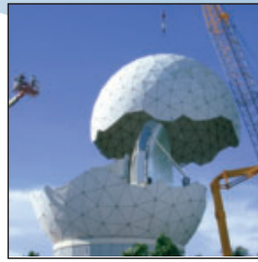
68-ft. (20.7 m) metal space frame radome top cap lift
