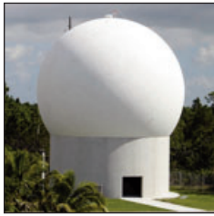
57-ft. (17.4 m) sandwich radome – weather
