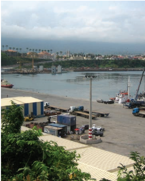
L-3’s integrated solution for West Africa includes a coastal surveillance network, infrastructure improvements and training to support its economic development strategy.
