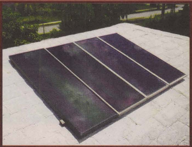
Figure 5 — Solar Panels. 60 watts of panels will allow you to run a pair of DC halogen lights all night without discharging the battery. Reserve is over a week!
