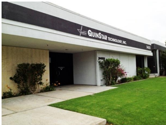
New additional facility at 3425 Lomita Blvd., Torrance
