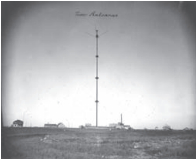
Fig. 2 – This photograph shows one of the two antennas erected by Fessenden in 1905 for the purpose of establishing a reliable transatlantic radio communications link. The installation in Scotland was destroyed in late 1906 by failure of a guy line. Insulators used to break up the guy lines can be plainly seen, as can the top loading “umbrella.” (Photo courtesy of the Office of Archives and History, Raleigh, North Carolina)
