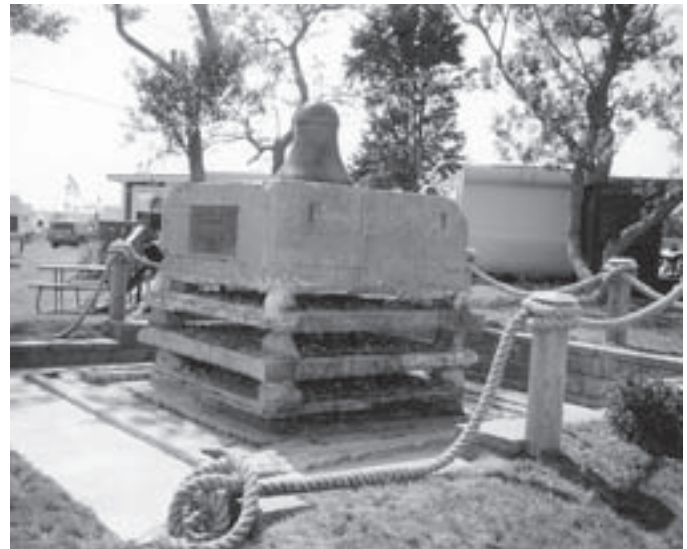
Fig. 4 – All that remains today of Fessenden's Brant Rock, Mass. 420-foot vertical radiator is this base unit. The lower portion of the ball-and-socket joint and the stacked insulating plates, along with some of the small cone-shaped insulators are visible in this photograph. The former NESCO laboratory site is now a park for house trailers and recreational vehicles. (Photo courtesy of Jay Ballard)
