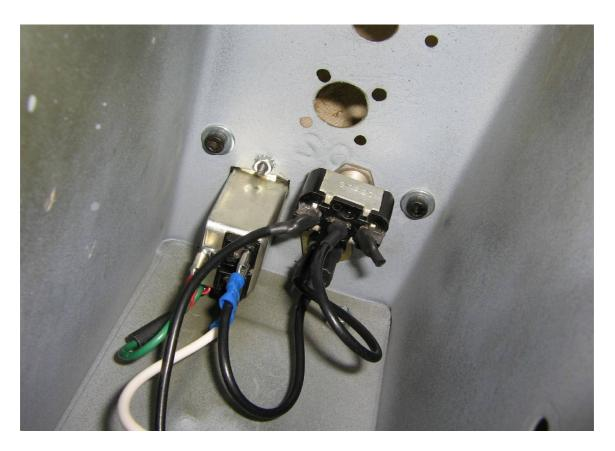
Rear view of the front panel AC power input connections.
