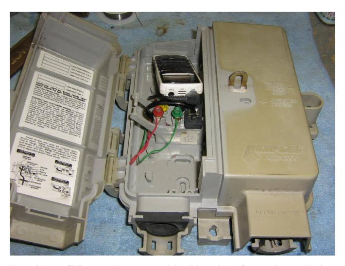
If you only have a Phillips screwdriver, you can only install the tap in the "Customer Access" side of the network interface box.
